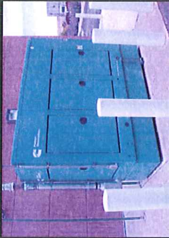
125 KW Back-Up Generator!
