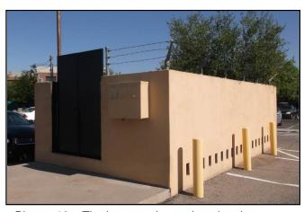
Picture 16 – The large enclosure housing the transformer north of the building.
