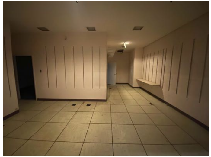
Computer room with raised floor.
