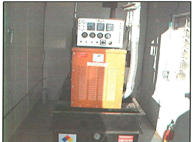
Picture 6 - South Portion – Emergency diesel generator and 210 gallon AST in American Tower™ equipment trailer.
