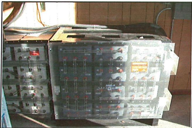
Picture 7 – South Portion – Lead acid batteries in American Tower™ equipment trailer.
